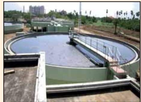
Sewage Treatment Plant
