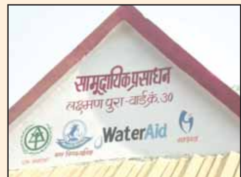
Community Toilet at Laxmanpura
