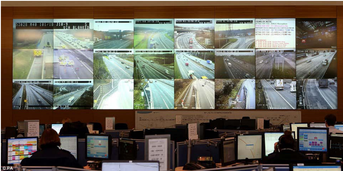
Figure 14: Operations Control Centre for Bus Operations. Courtesy: DIMTS
