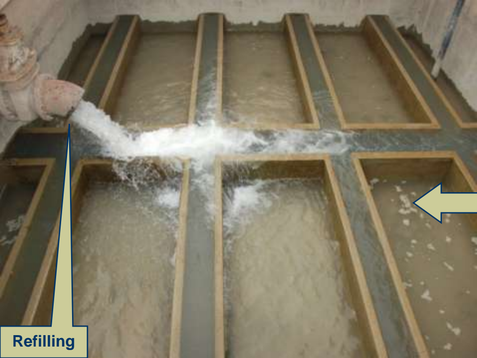
Lowering the Water Level up to the top Level of the Filter Bed
