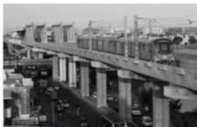
Much-awaited nod: The 14.6-km Phase II stretch, from Poonamallee to Vadapalani via Porur, received the final approval from the Commissioner of Railway Safety in May. S. JOTHI SANKARAN
