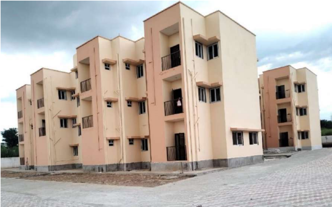
Completed DHP (Sports Hostel) under PMAY-U constructed by BMTPC using Prefabricated Sandwich Panel System – Quik Build 3D Panels at Bhalwal, Jammu, J&K
