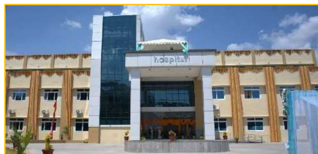
Family Quarters, SO's Mess, Hospital, Store Block & 180 Men Barrack at CRPF Group Centre, Jamshedpur
