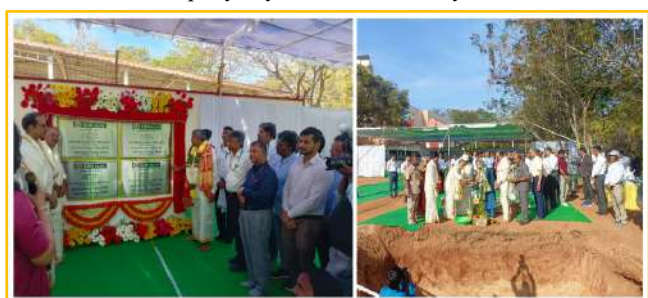
Foundation Stone and Bhoomi Pujan for the Additional Infrastructure works at IDBI Centre for Excellence in Banking & Finance (ICBF), Hyderabad performed by Shri Rakesh Sharma MD & CEO on January 24th, 2025.
