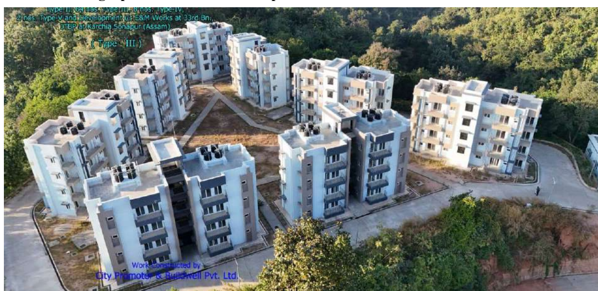
Residential Quarters 120 Nos. T-II, 64 Nos. T-III, 8 Nos. T-IV, 2 Nos. T-V at 33rd Bn., ITBP at Karchia, Sonapur (Assam)
