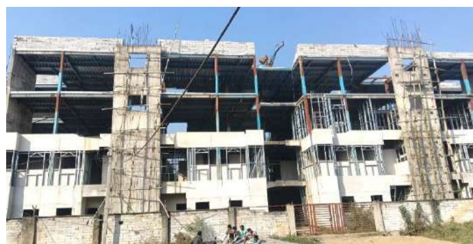
Demonstration Housing Project (for Contractual Safai Karamcharis) and Community Centre under PMAY-U being constructed by BMTPC using Light Gauge Steel Structural System – LGSF with V-infill Wall at Guwahati, Assam
