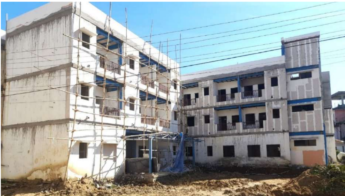
Demonstration Housing Project (Working Women Hostel) and Community Centre under PMAY-U being constructed by BMTPC using Prefabricated Sandwich Panel system – Flyash EPS(Beads) Cement Sandwich panels at Dimapur, Nagaland
