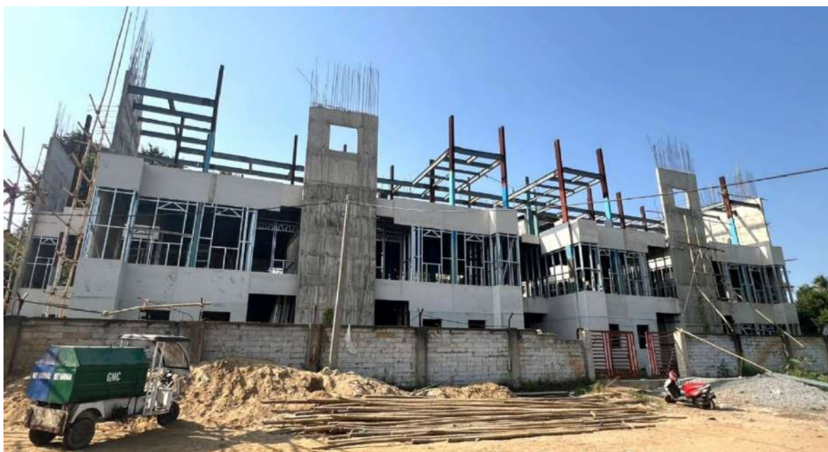
Demonstration Housing Project (Contractual Safai Karamcharis) and Community Centre under PMAY-U being constructed by BMTPC using Light Gauge Steel Structural System – LGSF with V-infill wall at Guwahati, Assam
