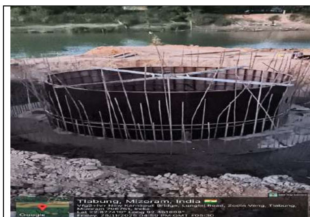
Bridge over river Karnaphuli in Mizoram
