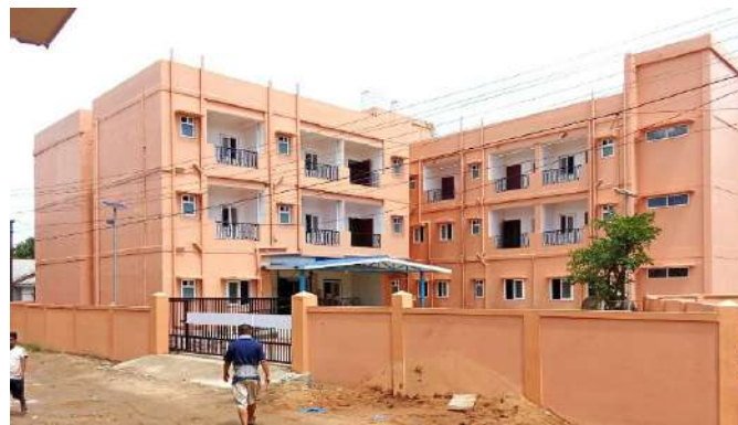
Demonstration Housing Project (Working Women Hostel) and Community Centre under PMAY-U constructed by BMTPC using Prefabricated Sandwich Panel System –EPS Cement Sandwich Panels with Steel Structure at Dimapur, Nagaland
