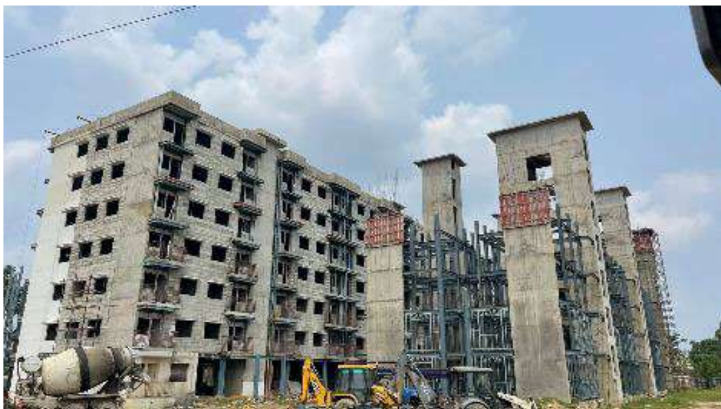
Ongoing LHP at Agartala, Tripura
