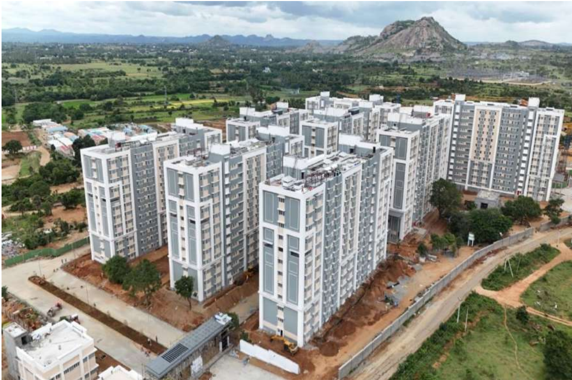
Affordable Rental Housing Complex in Hosur, Tamil Nadu constructed by M/s Vidiyal Residency Pvt Ltd. for industrial workforce of Tata Electronics Pvt Ltd+, offering 10,756 dormitory beds in 2,700 rooms
