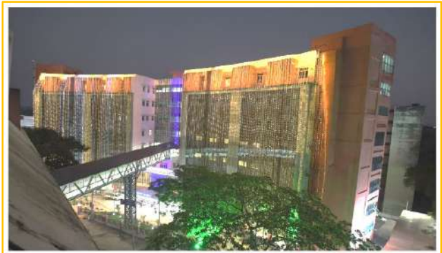
PMSSY Block, Pay Ward, Connecting Bridge & Multi Level Car Parking at SCTIMST, Thiruvananthapuram
