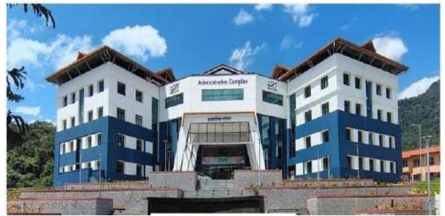
Administrative Complex Building at Indian Institutes of Science Education and Research, Vithura, Thiruvananthapuram
