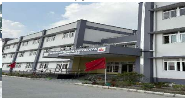
‘A’ Type School Building at Udalguri, Assam
